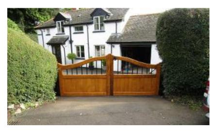
The scheme is utilising the EA's PFR framework with the contractor, Watertight International, utilising timber gates that are British Standard Kitemarked to give the village passive flood protection. Installation of the PFR measures is due to be completed prior to April 2022.
